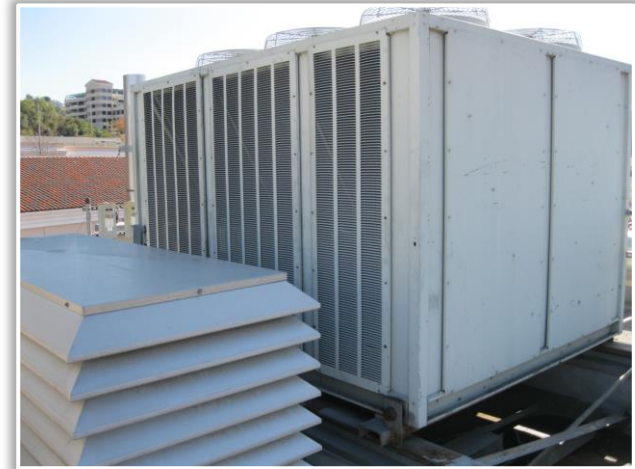
Aging Dx condenser unit at Arroyo Seco that will be eliminated (total of 7 -9 Dx systems will be eliminated across campus through central plant expansions)
